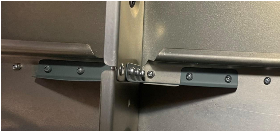
Figure 9 - Both Clips Installed
