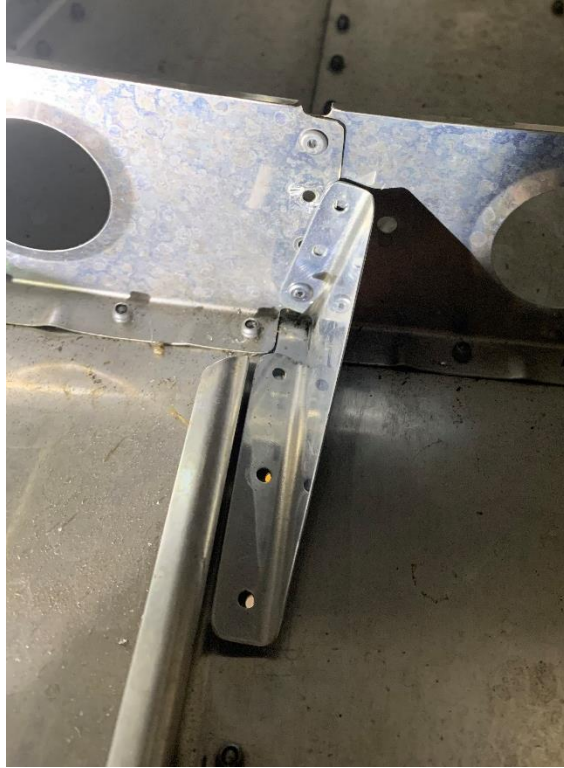
Figure 8 - Riveting Lower Hole
