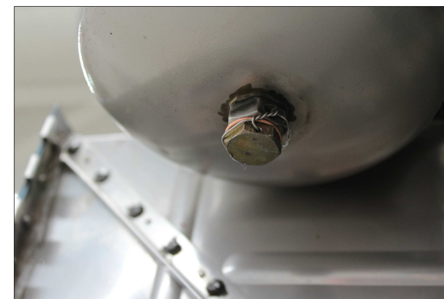
FIGURE 5: SAFETY WIRE OIL TANK DRAIN PLUG
