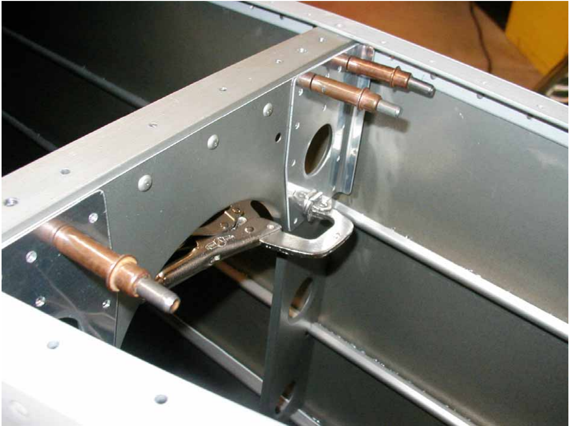
Doublers clecoed/clamped in place after match drilling.
