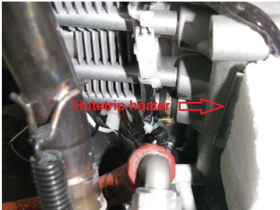
FIGURE 3: INSTALL CRANKCASE HEATER
