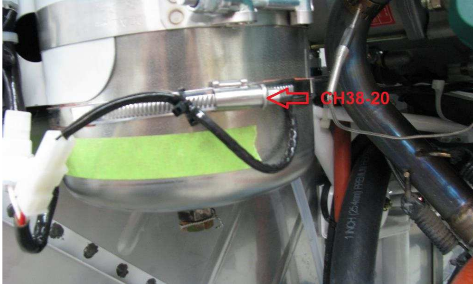
FIGURE 2: INSTALL TANK HEATER
